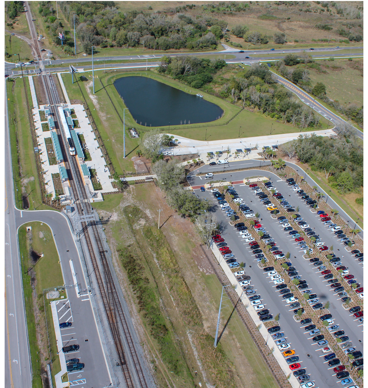
Poinciana SunRail Station
